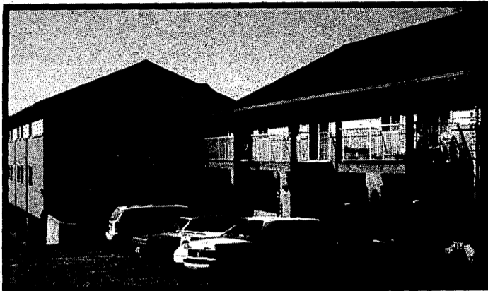
SOUTH CAMPUS PLACE 2600-2608 Douglas Ave., Bellingham, WA 98225
