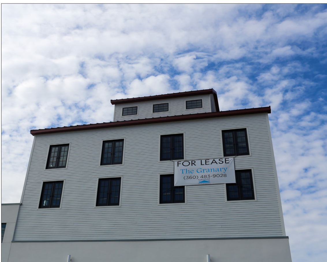
Waterfront construction is expected to be complete by fall 2020.
