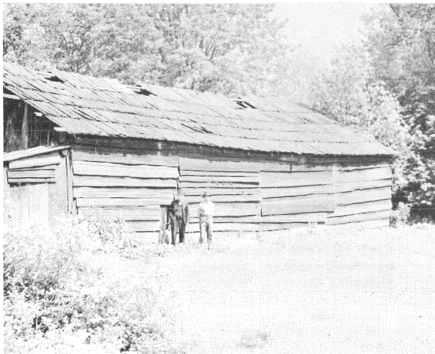
Fig. 12. Smoke holes are visible in this photo and appear to indicate three fires were used by the inhabitants. The longhouse was built circa 1850. (Jeffcott Collection)
