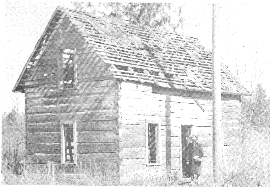
Figure 30. Tom Nicklin home, Roeder (near Everson) shows the overall construction of a dove-tail home. (Jeffcott Collection)
