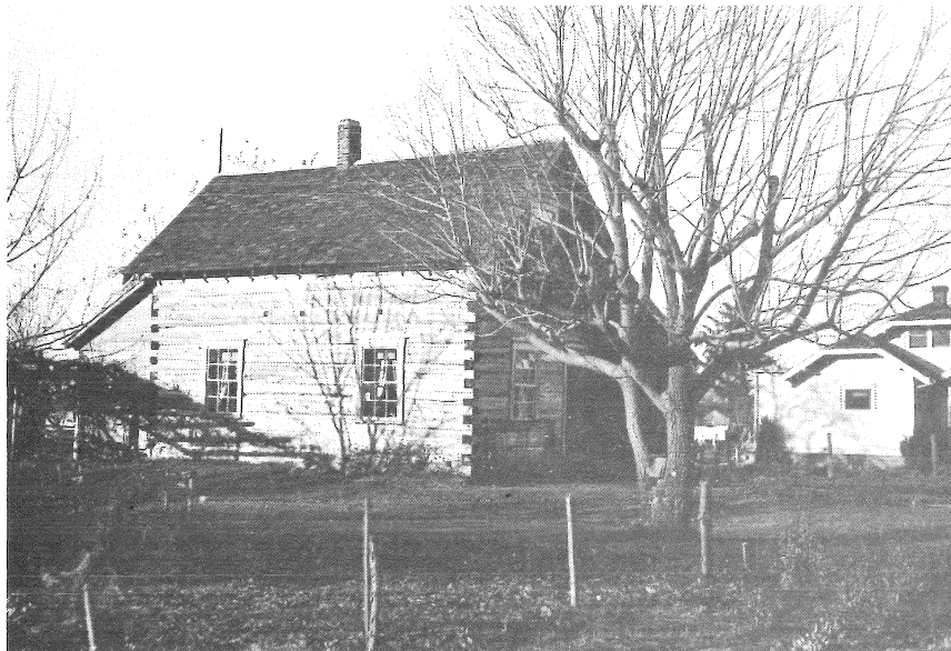
Figure 24. The original Slade home in Lynden, also built of alternating tier and square-notch construction. Note the lean-to additions. (Jeffcott Collection)
