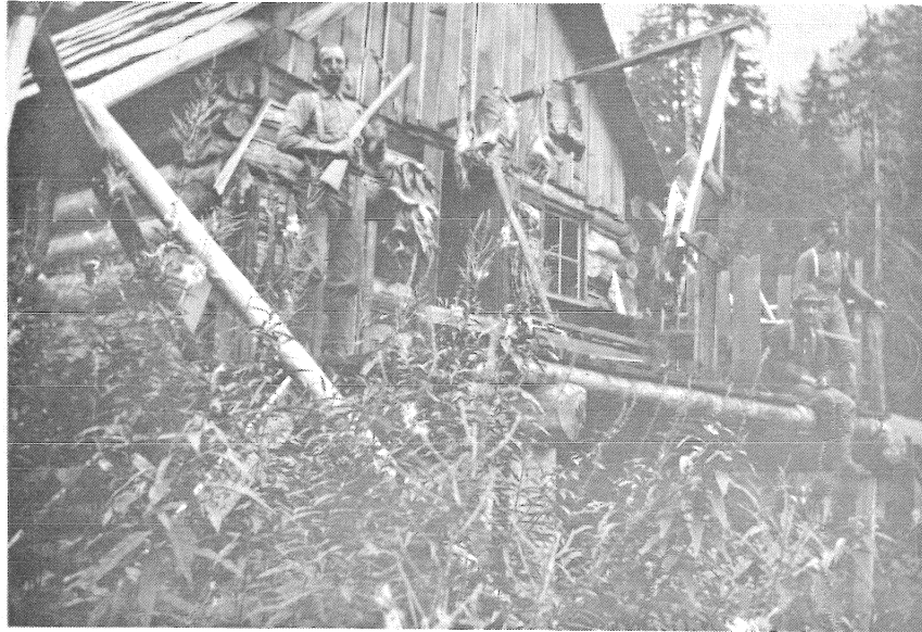
Figure 35. V-notch construction is evident in this early photo. (Whatcom Museum)
