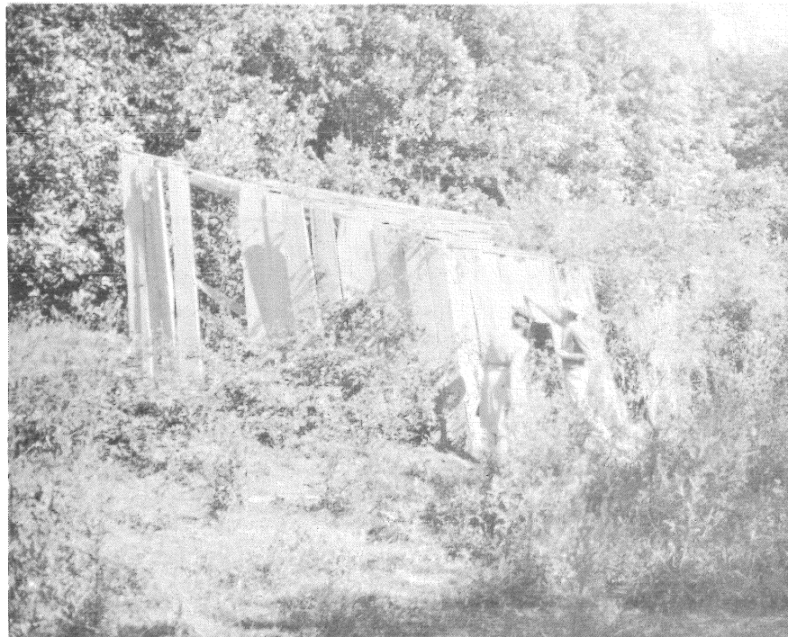
Fig. 3. Remains of a Lummi Indian shed-roof house at Old Lummi Village circa 1945. Note the vertical siding, pitch of the roof, and entrance. (Jeffcott Collection)
