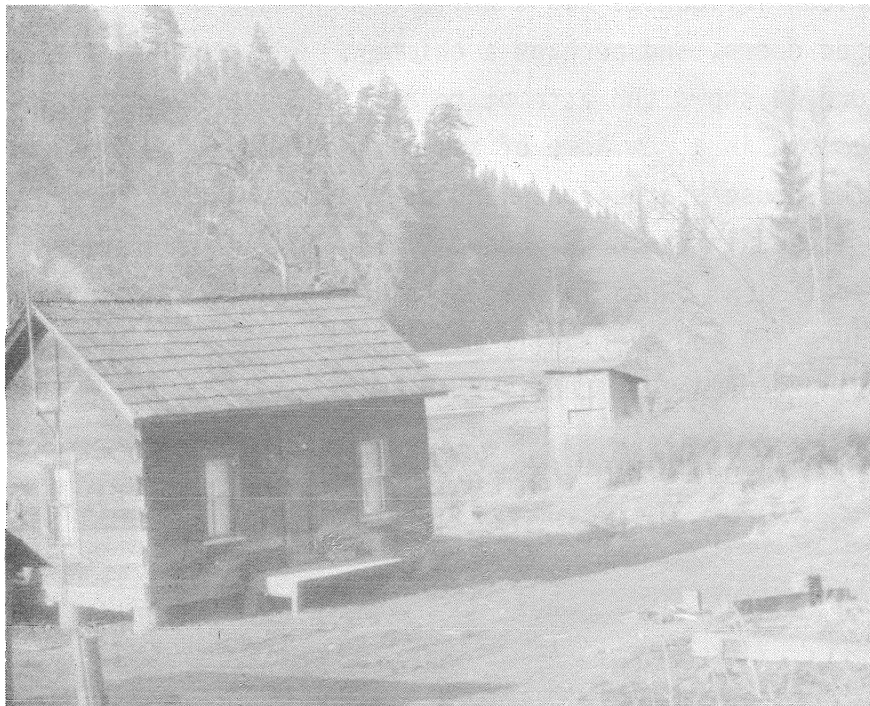
Figure 15. Nooksack Indian home near the Forks, built circa 1880, is a dove-tail log cabin (Jeffcott Collection)
