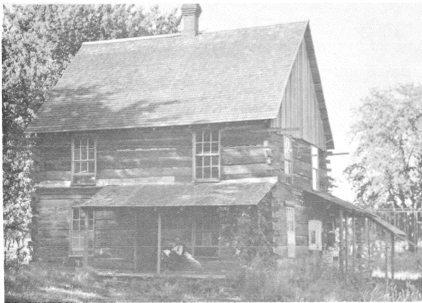
Figure 27. Square-notched log cabin of Bill Johnson who settled near Hopewell. Note the porch additions, steep roof and central chimney. (Jeffcott Collection)
