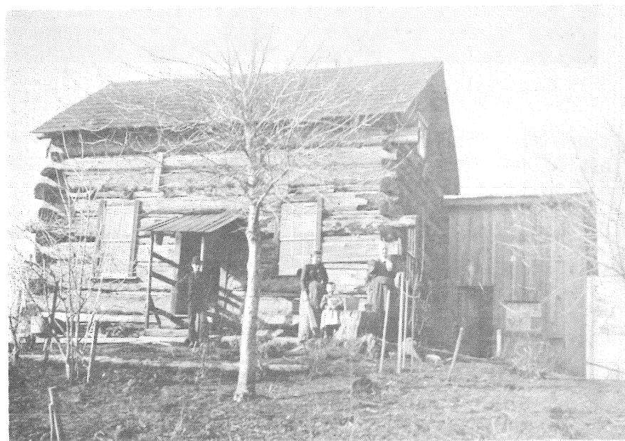
Figure 26. The George Bremner home, built in 1880. The square-notches extend at the corners; a lean-to has been added. This home served as the first Delta post office. (Jeffcott Collection)
