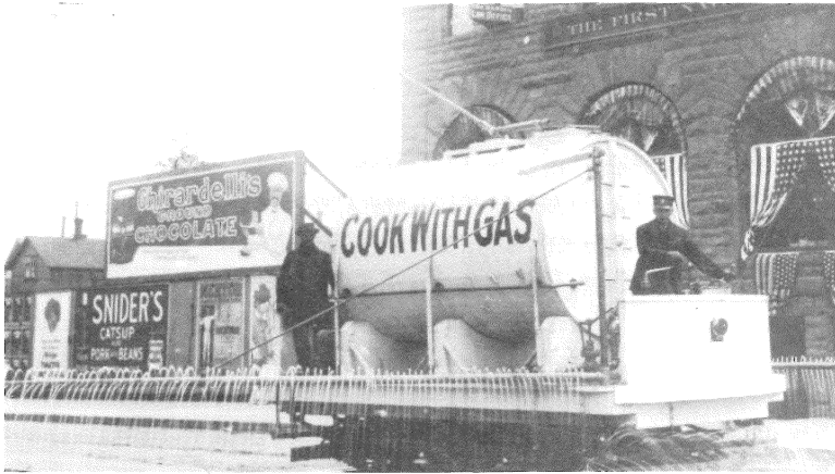
Figure 18. The highly successful sprinkler car which went into service in 1908. (Puget Power Collection, CPNS)
