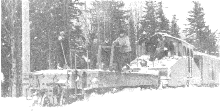
Figure 33. Locomotive #250 and the express car team up to traverse the Pacific Northwest Traction line after the blizzard of 1916. (Puget Power Collection, CPNS)
