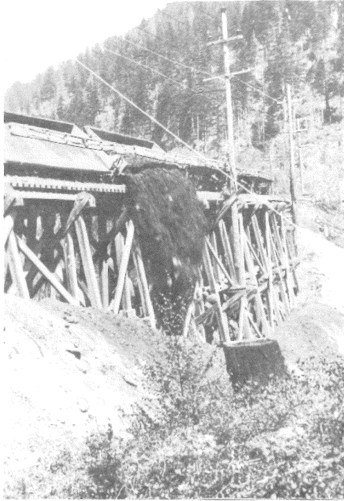
Figure 36. Part of Pacific Northwest Traction's 1921 trestle filling operation: the Gravel Pit fill between Chuckanut and Wildcat Cove. (Puget Power Collection, CPNS)
