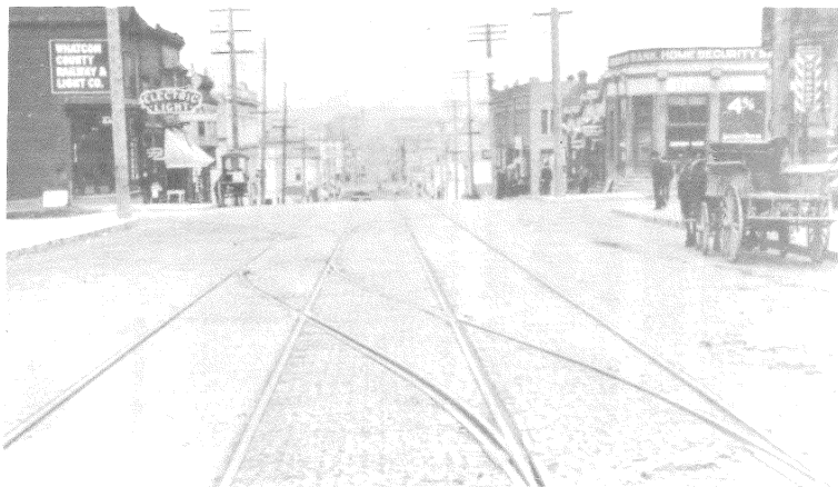
Figure 14. A 1908 view of the intersection of Holly and Bay. The headquarters of Whatcom County Railway and Light are at the left. (Puget Power Collection, CPNS)
