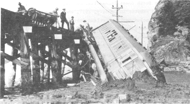
Figure 47. The derailment of car #75 at Rocky Point in September, 1928. (Puget Power Collection, CPNS)
