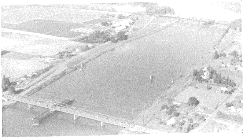
Figure 52. Concrete pilings are the only remnants of the Skagit River bridge built by Pacific Northwest Traction. (Photograph by Author)
