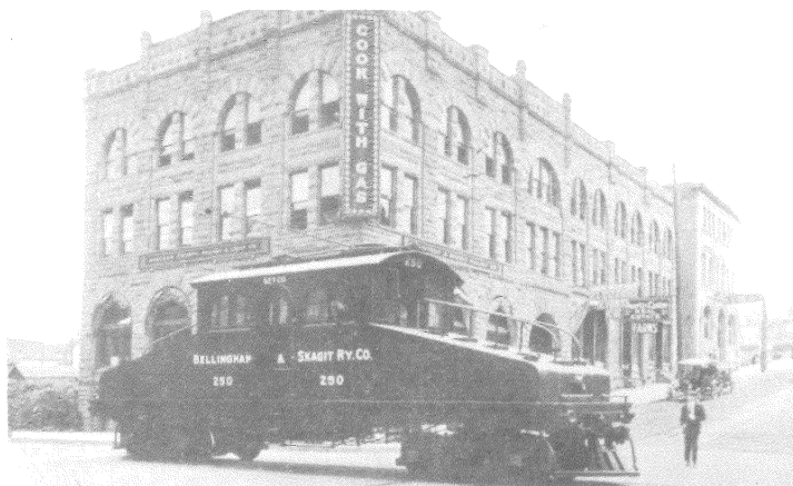
Figure 30. The new freight locomotive, #250, in front of the Pike Building at Holly and Elk. (Puget Power Collection, CPNS)
