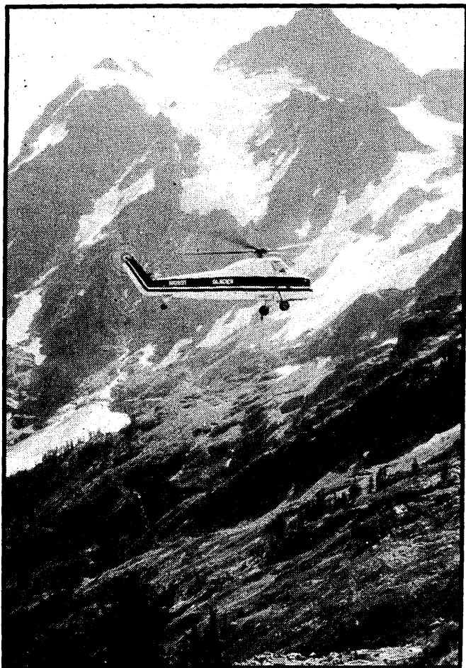
Helicopter transports concrete to top tower of new chair.
