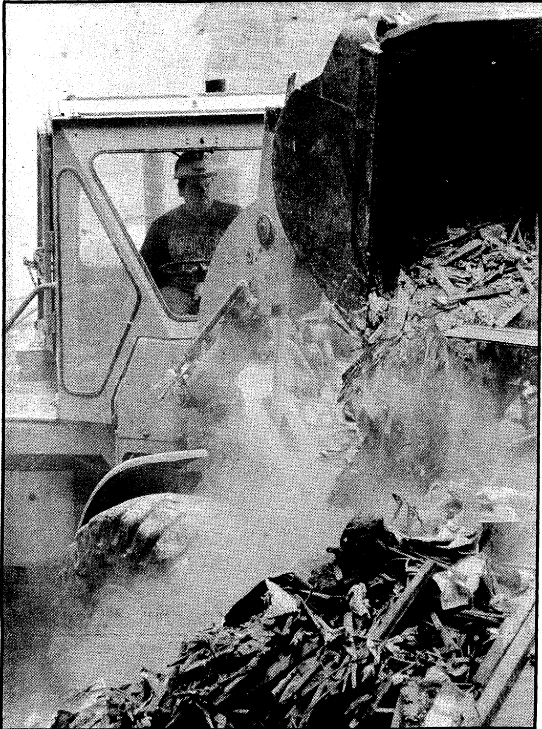
Construction worker plows debris by Edens Hall.
