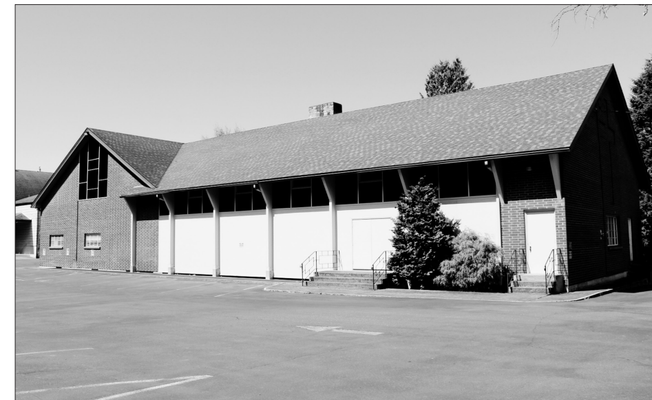
Located on 910 N. Forest St., the Seventh-day Adventist Church is selling their property, which could potentially cater to student housing, depending on the developer. // Photo by Melissa McDonough
