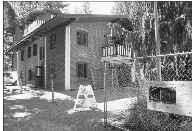
Ridgeway Kappa is set to open back up Tuesday, September 15. The renovated building will include updated plumbing and a new fire alarm and sprinkler system. // Photo by Alexandra Bartick
