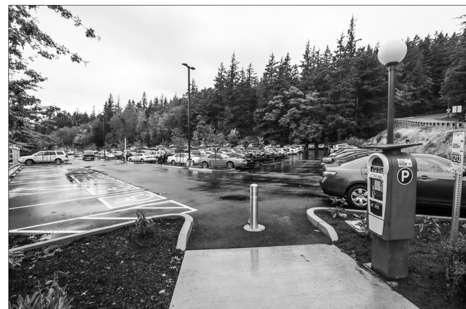
The commuter parking lots were paved over summer as part of a parking construction project. // Photo by Katie Webber
