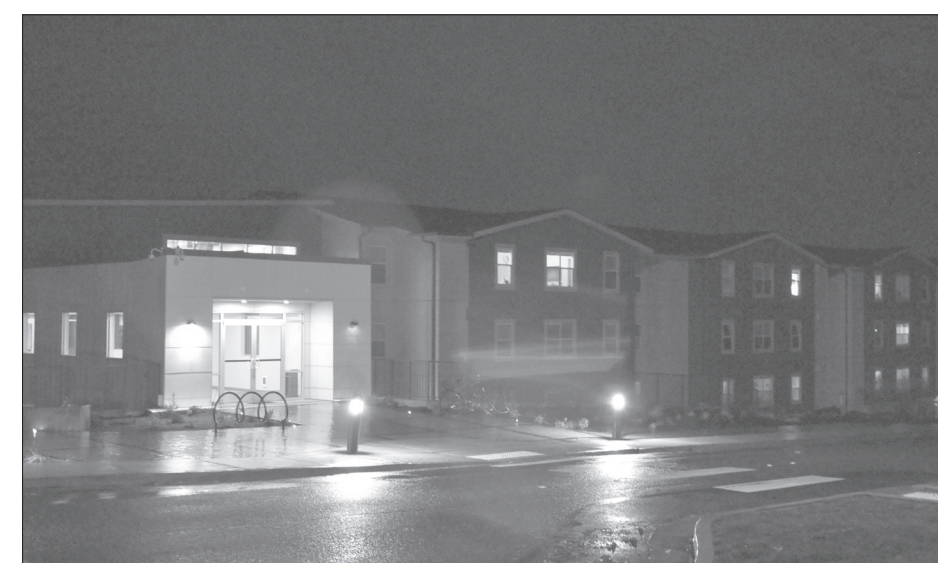
Gather Bellingham opened at the end of September this year. Students speculate its hasty construction to open for fall led to unaddressed safety issues. // Photo by Kirstyn Nyswonger
