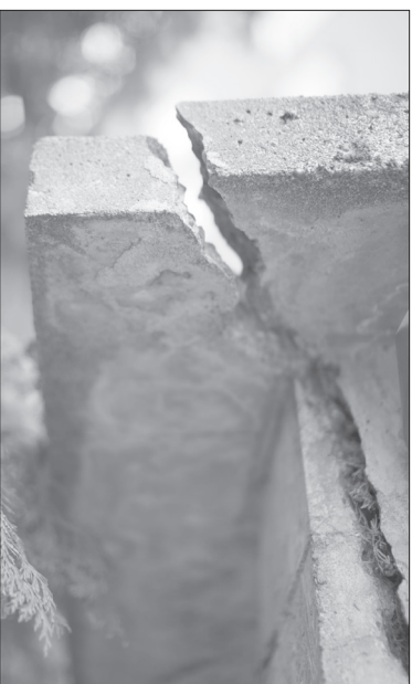
Crack in foundation of campus building. // Photo by Mathew Roland
