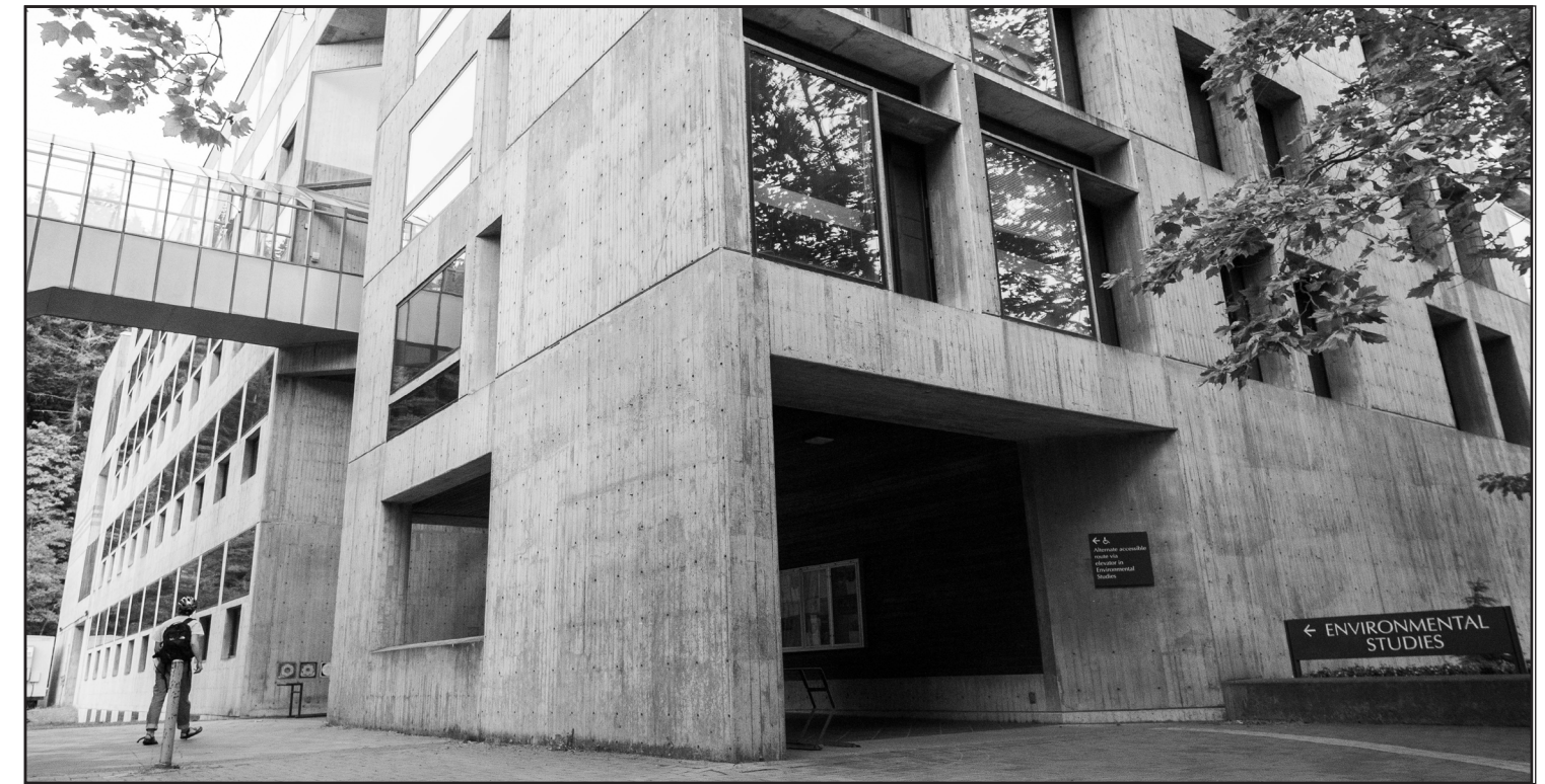
A photo of the outside of the Huxley building where the environmental studies department is located taken June 26, 2019. // Photo by Mike Oh
