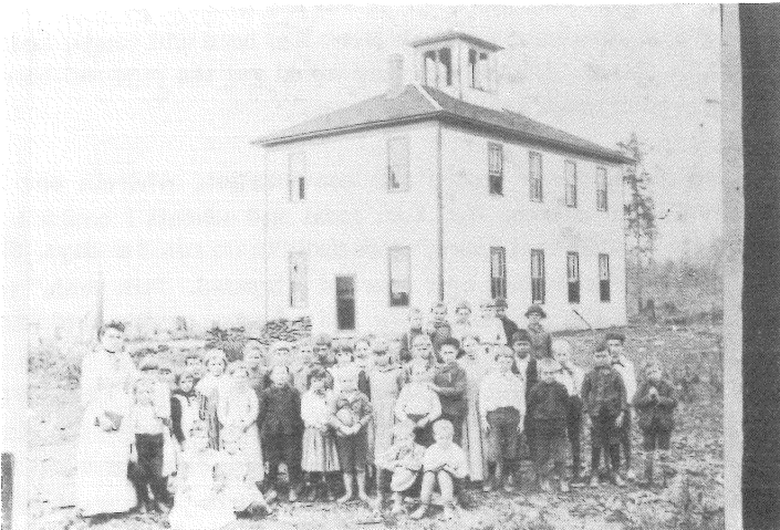
Figure 9. Bay View's Three-room Schoolhouse, Second Structure, early 1900s.
