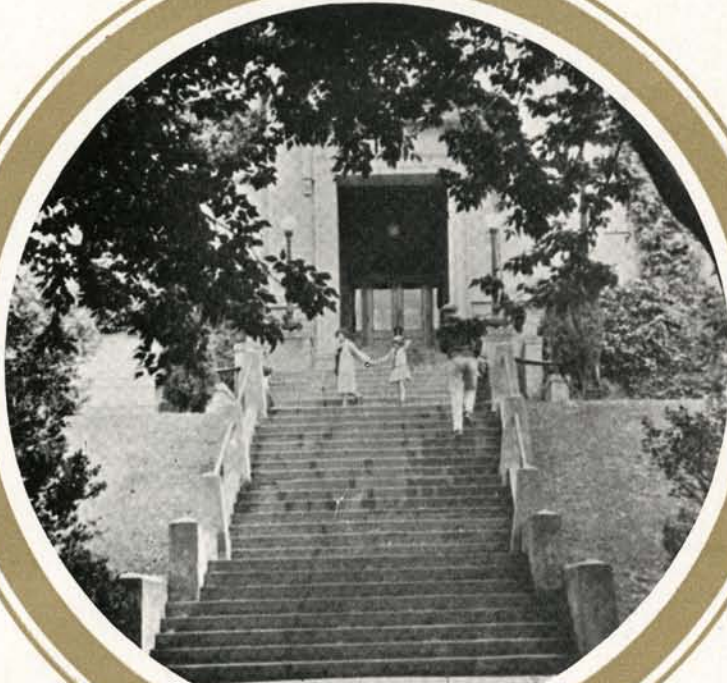
Steps to the main Entrance
