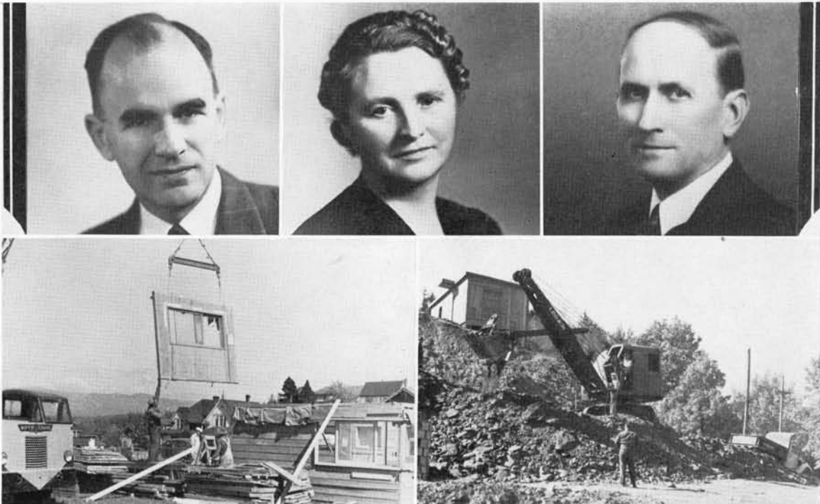
THE TRUSTEES: Joseph T. Pemberton, Mrs. Violet Boede, and Vern Branigin. Appointed by the Governor, this board formulates and appraises details of finances, building, and general policy. LEFT: The Sehome housing project moves in. RIGHT: Cleared away for the new men's dorm location were the College Inn and half a hill.
