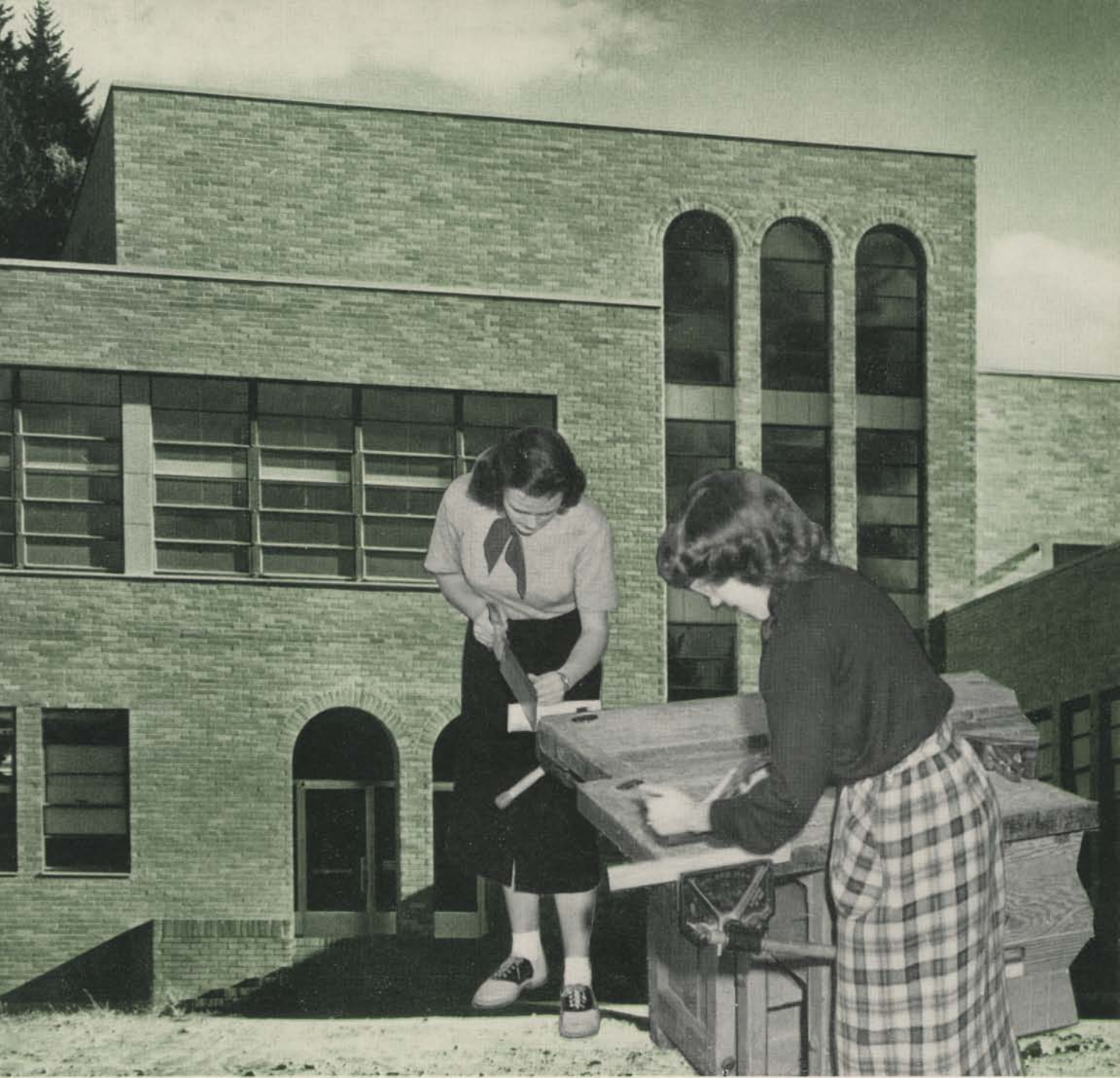
Industrial Arts Building
