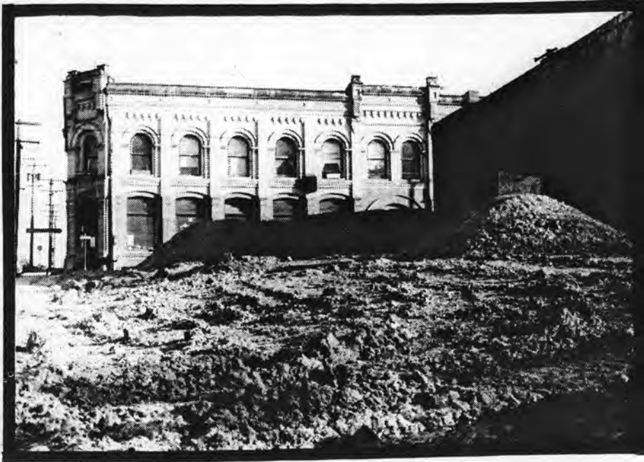
After the Bulldozer: where our co-op garden was, subsoil and gravel---soon a cyclone fence.
