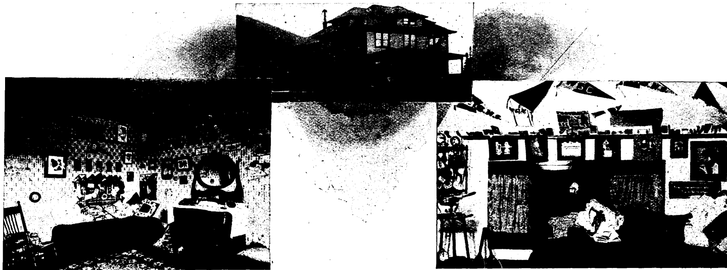
VIEWS OF THE OUTSIDE AND FROM THE SECOND AND THIRD FLOORS OF THE DORMITORY
