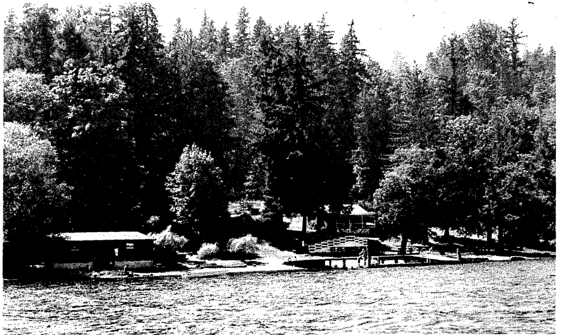
Improvements on Lakewood, student-owned property on Lake Whatcom, have been halted due to a lack of funds.
