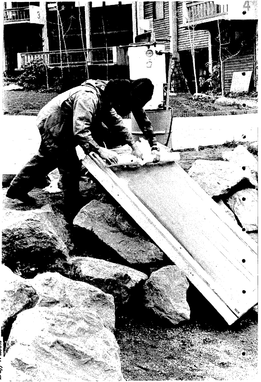
HERE COMES THE SUN — The heating panel of a solar-powered water heater is given an extra layer of protection. The device raised the temperature of part the water up 20 degrees on Saturday, with clouds in the sky and a chill in the air. The solar-powered water heater was built last summer for the King County Fair and appeared at the Second Annual Futures Fair.
