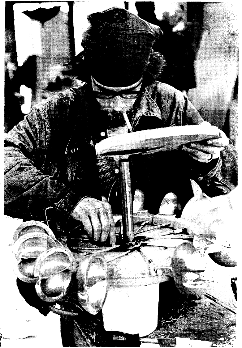
BUILDING A WATER WHEEL — P.F. "Rocky" de Armond builds a Pelton wheel Saturday at the Futures Fair. The wheel is equipped with 15 aluminum "buckets" to receive jets of water and, in turn, generate energy.
