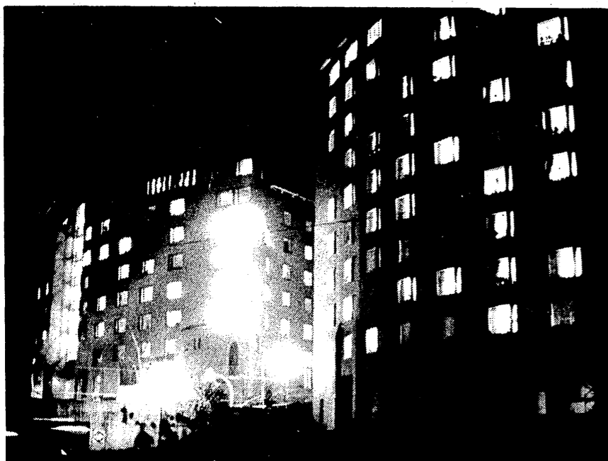
IN A BROWNOUT, electrical output in Western's dorms would be reduced.
